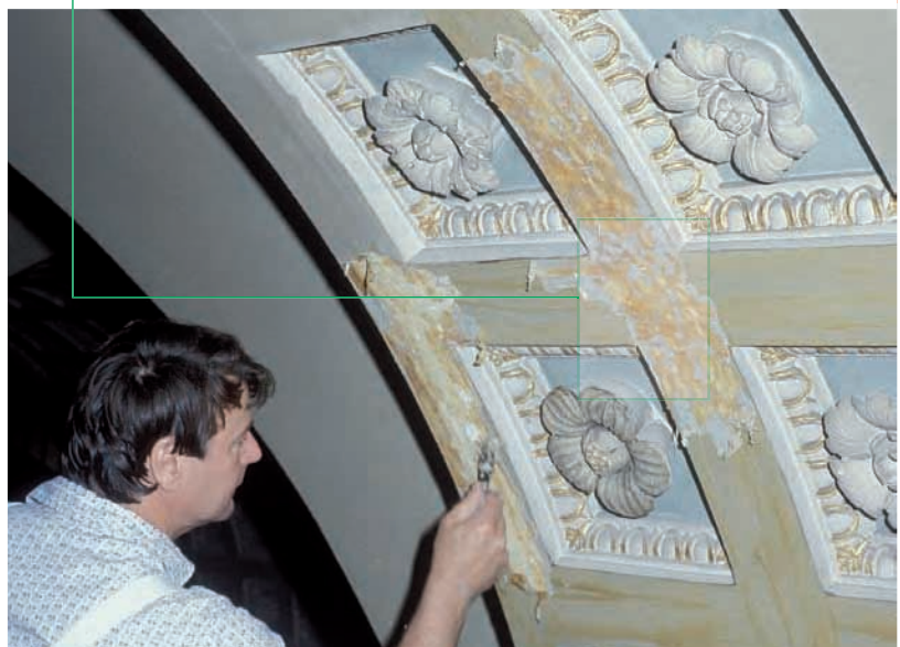
Photo Scheidel: Semper Gallery Dresden – m.a.c.s.® SG 94 Paint Stripper in application
